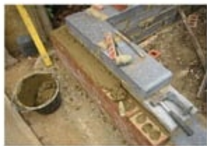
Laying bricks with Portland cement mortar
